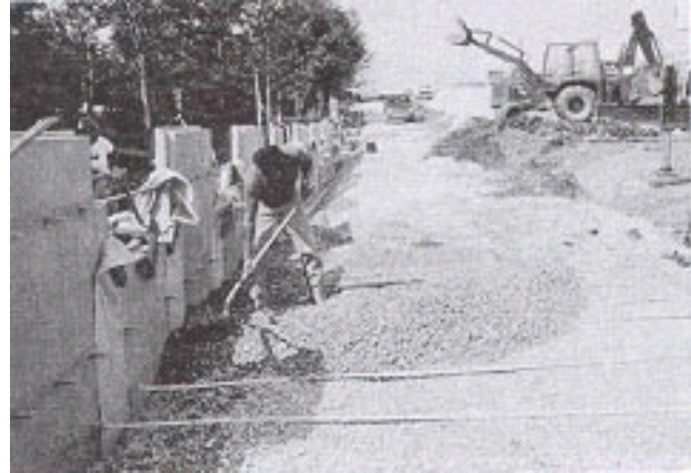
Construction of MSE wall
