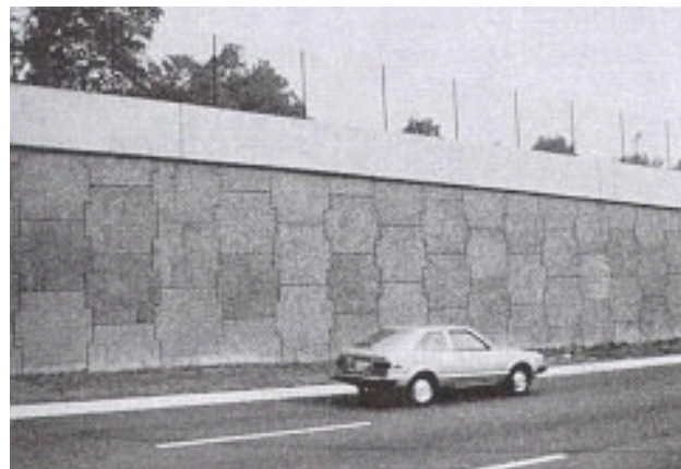
Completed MSE wall
